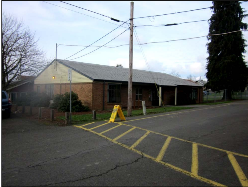
Sec. 1.01 – View to northwest of south elevation at left and east elevation at right.
